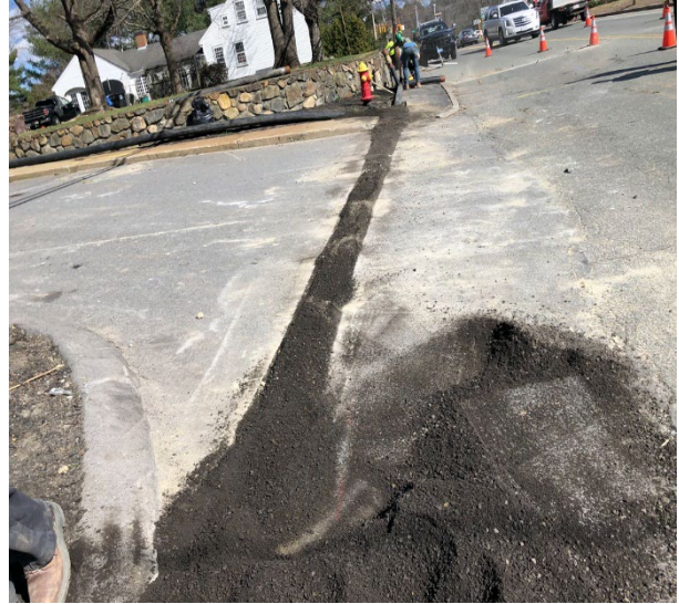
Photo 2: Excavation and Burial of Bypass Pipe
