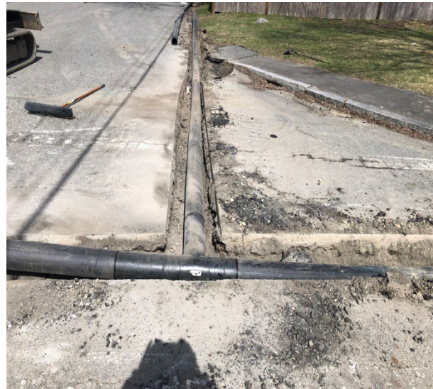
Photo 4: Bypass Pipe Installation
