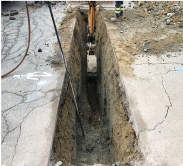
Photo 1: Test Pit Excavation on Southfield Drive
