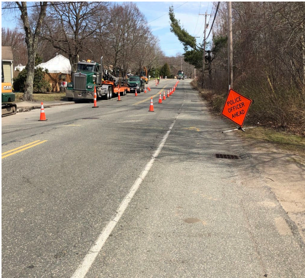
Photo 3: Traffic Controls on Auburn Street
