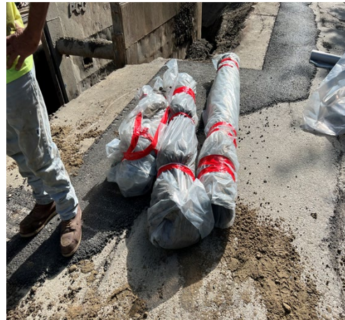
Photo 4: Removal and Disposal of 6" Asbestos Pipe
