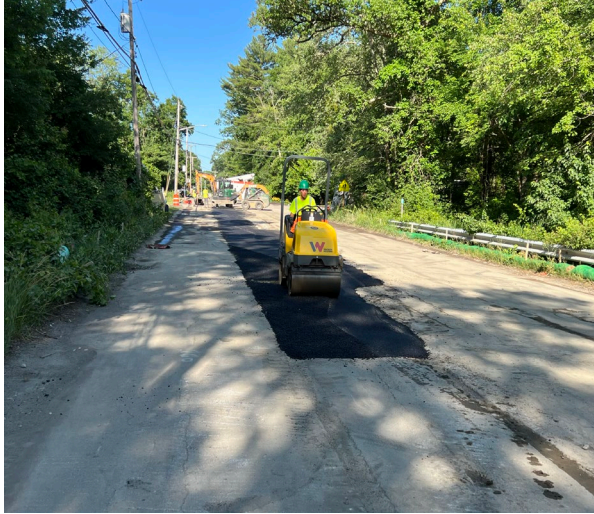
Photo 1: Trench Compaction After Paving
