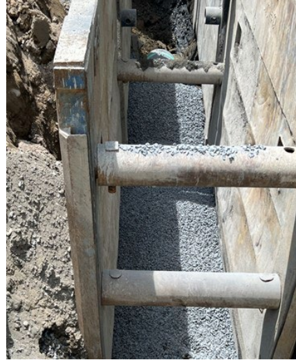
Photo 2: Crushed Stone Placed After Pipe Installation
