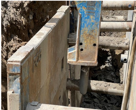
Photo 3: Rock Breaking via Hammer
